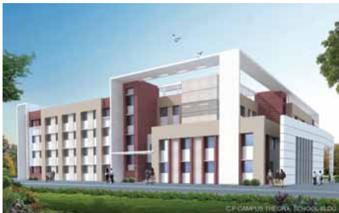
School Building Career Point Residential Campus, Thegda
