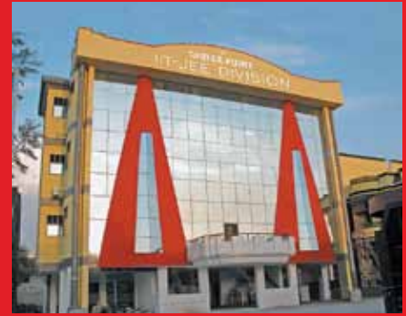
128 Shakti Nagar (Academic Building-1, Centrally Air Conditioned)
